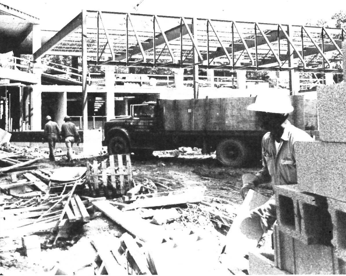
Steel framing is now being added to the already existing concrete frames.
